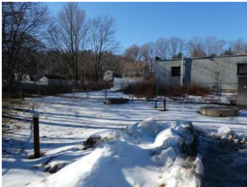
Figure: Thermal Treatment Area on Southern Side of Valley Manufacturing Building (Fourth Five-Year Review)
